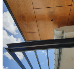
8 PREFINISHED STAINED & TREATED EXPRESSED JOINT PLYWOOD SOFFIT
