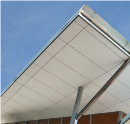
7 PAINT FINISH EXPRESSED JOINT FIBRE CEMENT SOFFIT
