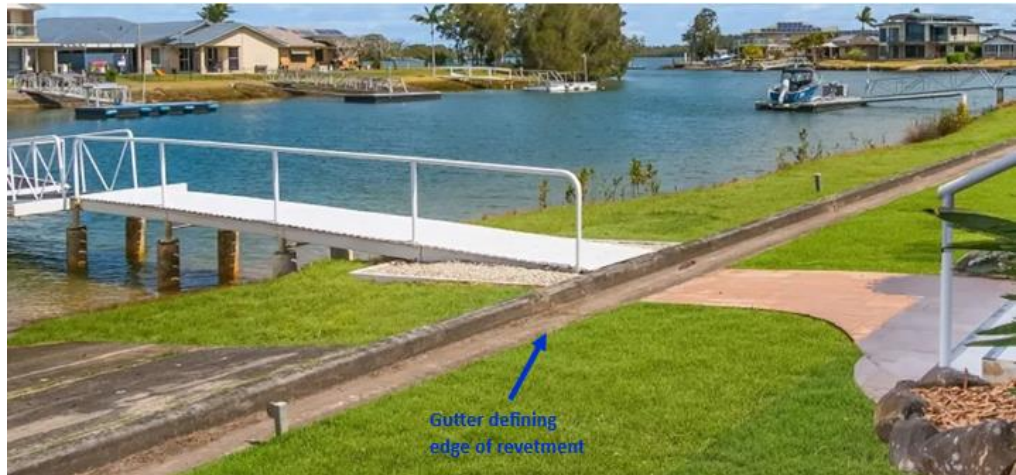
Photo – Edge of revetment in Ballina Quays estate.
