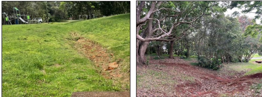
Plate 20: Drainage channels are eroding and require protection and edge plantings.
