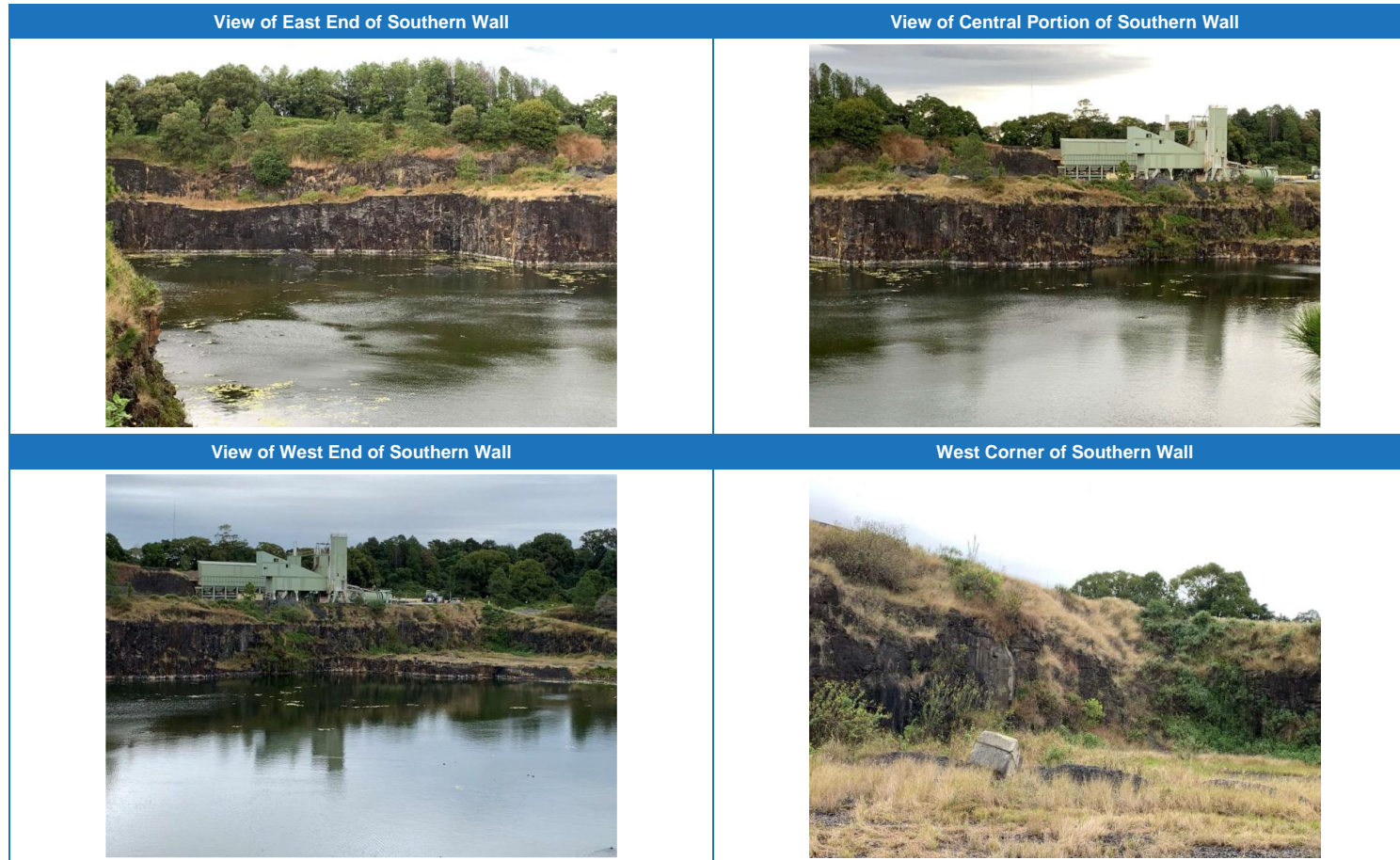
Figure B. 7. Southern Wall (1 of 2)
