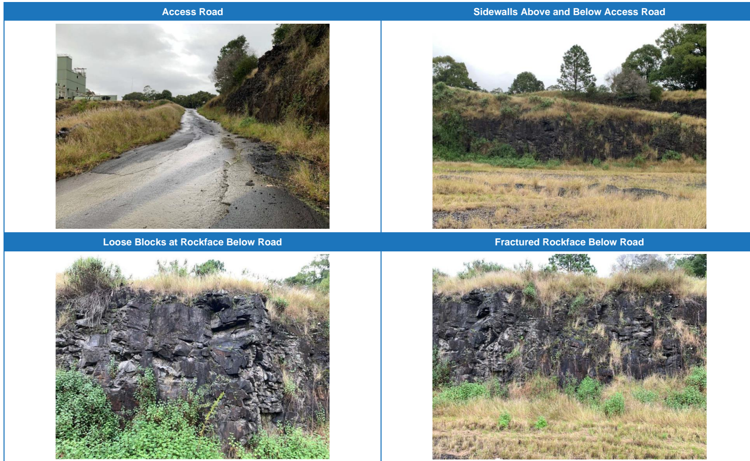
Figure B. 6. Access Road at Southwest Corner of Void (2 of 2)
