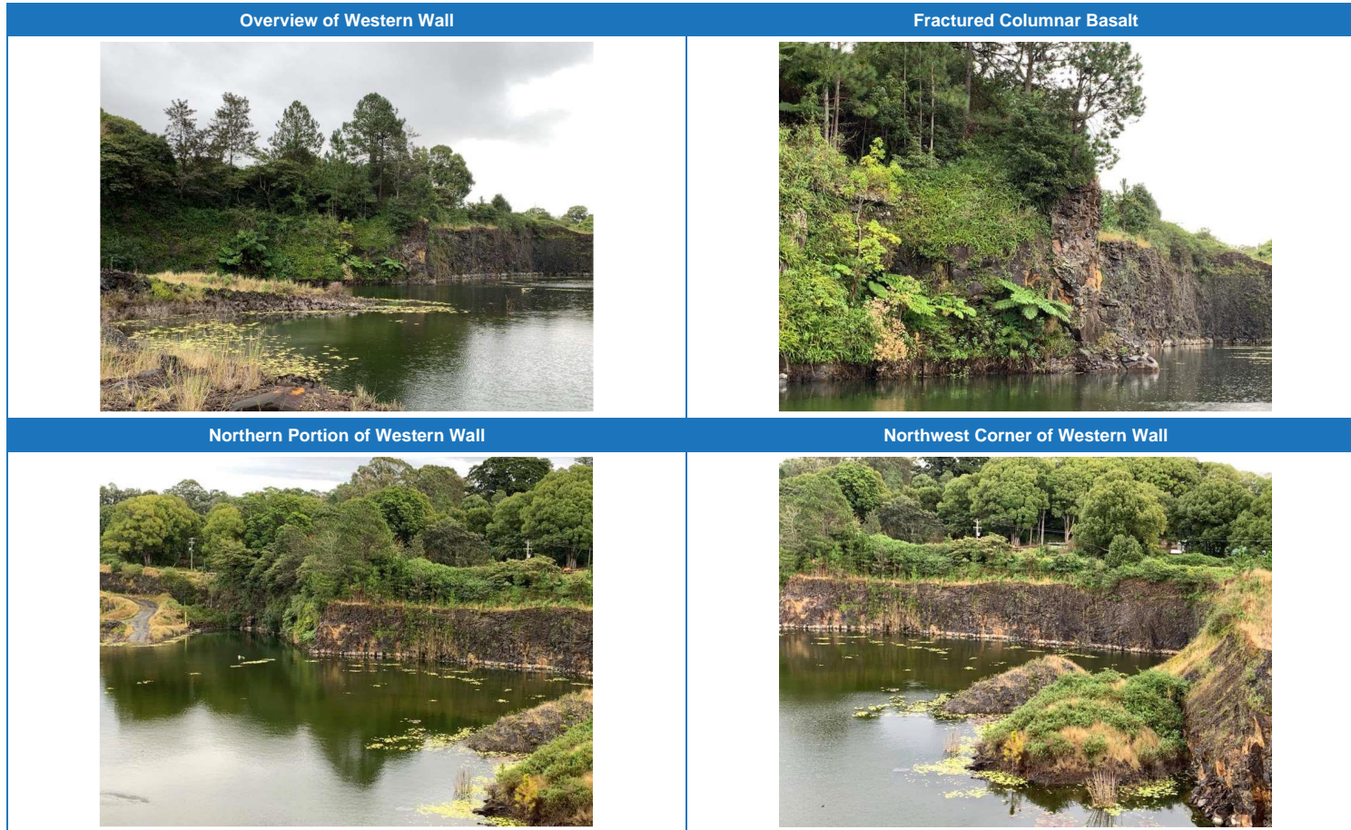
Figure B. 4. Central to Northern Portion of Western Wall (2 of 2)
