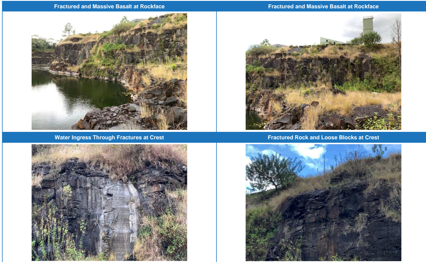
Figure B. 8. Southern Wall (2 of 2)
