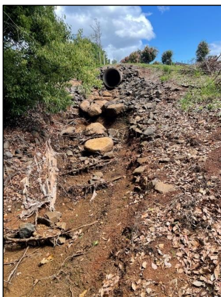
Plate 30: The stormwater channel from Elvery Lane requires rock lining (left) and the northern bank area (right).
