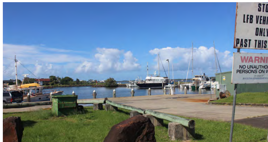
O existing concrete wharf at the harbour
