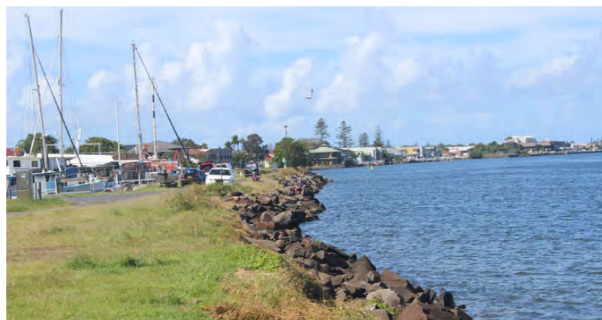
P south wall to the harbour, adjacent to the Richmond River
