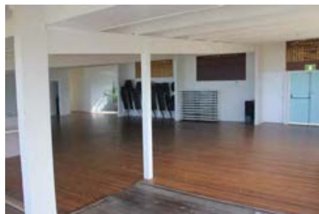
Main hall - sagging beams and trip hazards between flooring materials
