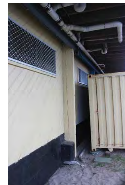
Signs of cracking in support columns / exposed sewer pipes
