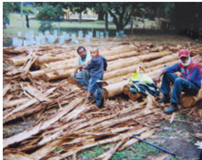
Preparing timber for the boardwalk, Cabbage Tree Island, 2010. Photo by Marcus Ferguson
