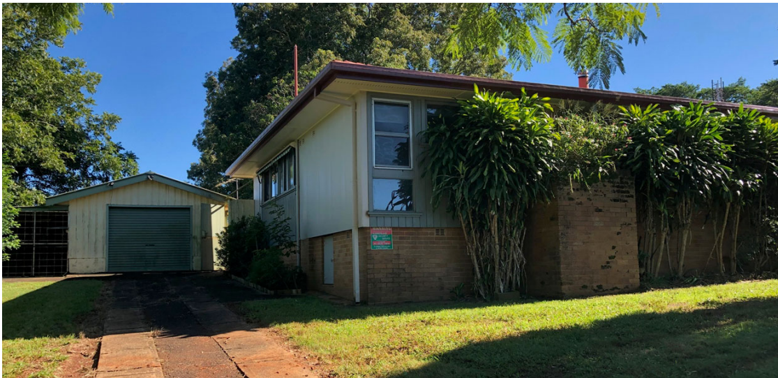
Photo 1 – Existing dwelling and garage at 46 Lindendale Road, Wollongbar
