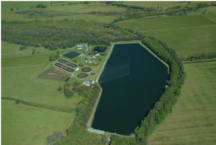
Existing Ballina Sewage Treatment Plant
