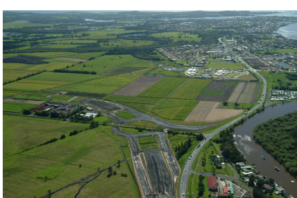
Earth works pre-loading associated with future Tevan Rd interchange
