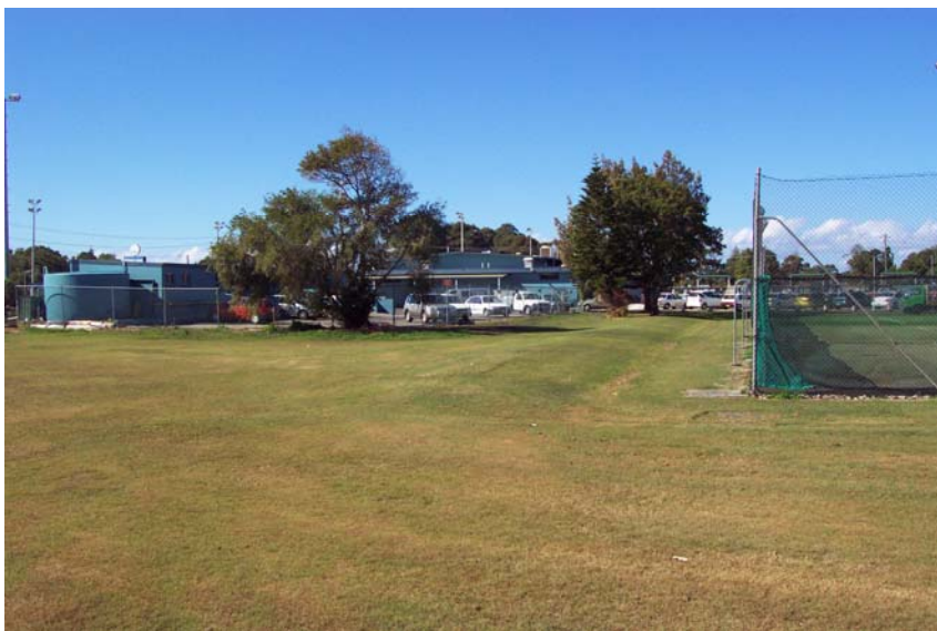
Photo 23 – Easterly view of drainage area between the Tennis Courts and the Bowling Club car park.
