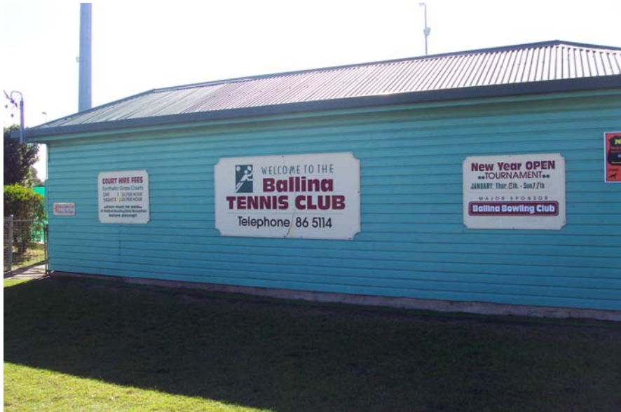
Photo 3 - Tennis Shelter viewed from Burnet Street.
