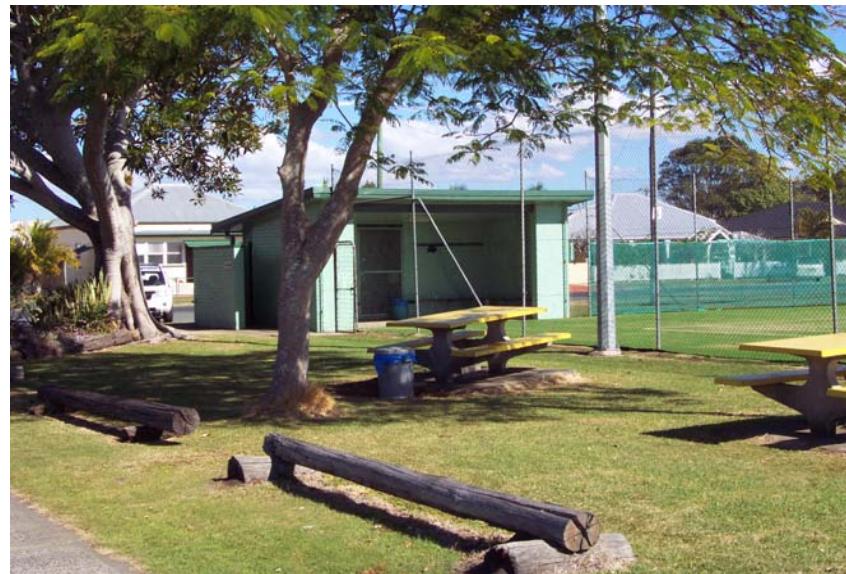
Photo 10 – Amenities & tennis shelter with Burnet St in background.
