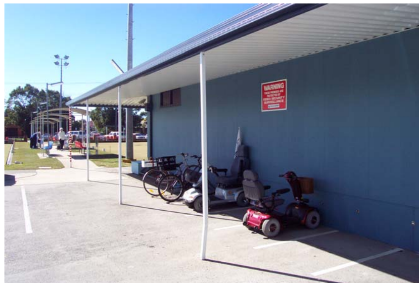
Photo 32– Western wall of Bowling Club viewed from car park.
