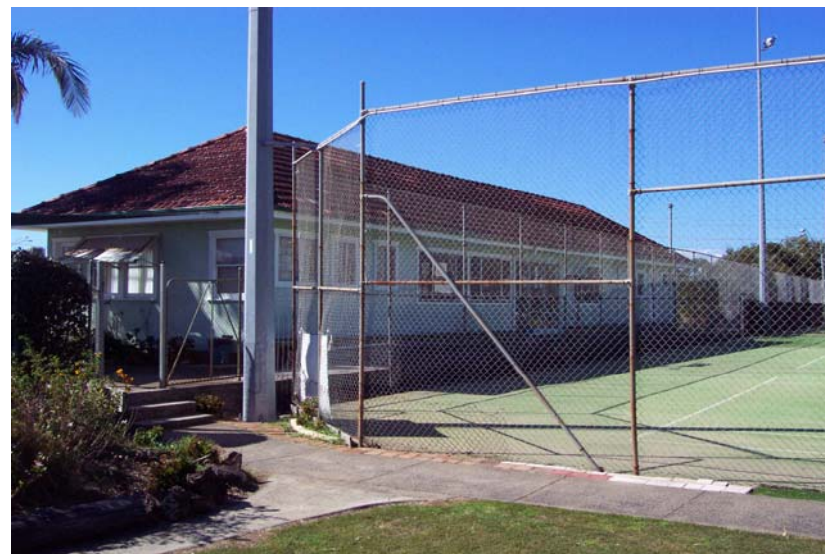
Photo 8 – Tennis Club House view from internal access.
