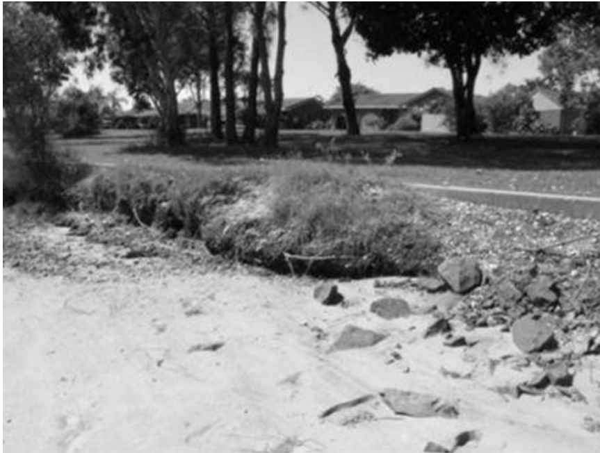
Plate 9: Area of erosion at Prospect Lake.
