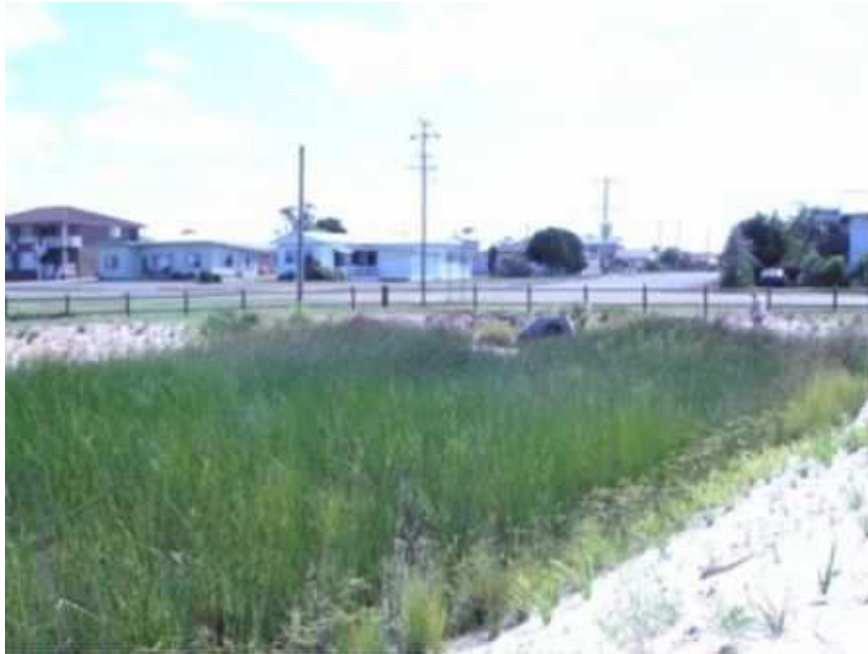
Plate 11: Example of a constructed stormwater wetland in a residential situation (location: Evans Head, NSW)
