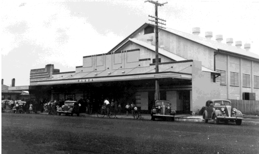
Plaza Theatre, River Street, Ballina, showing art deco facade. Image courtesy of Richmond River Historical Society.
