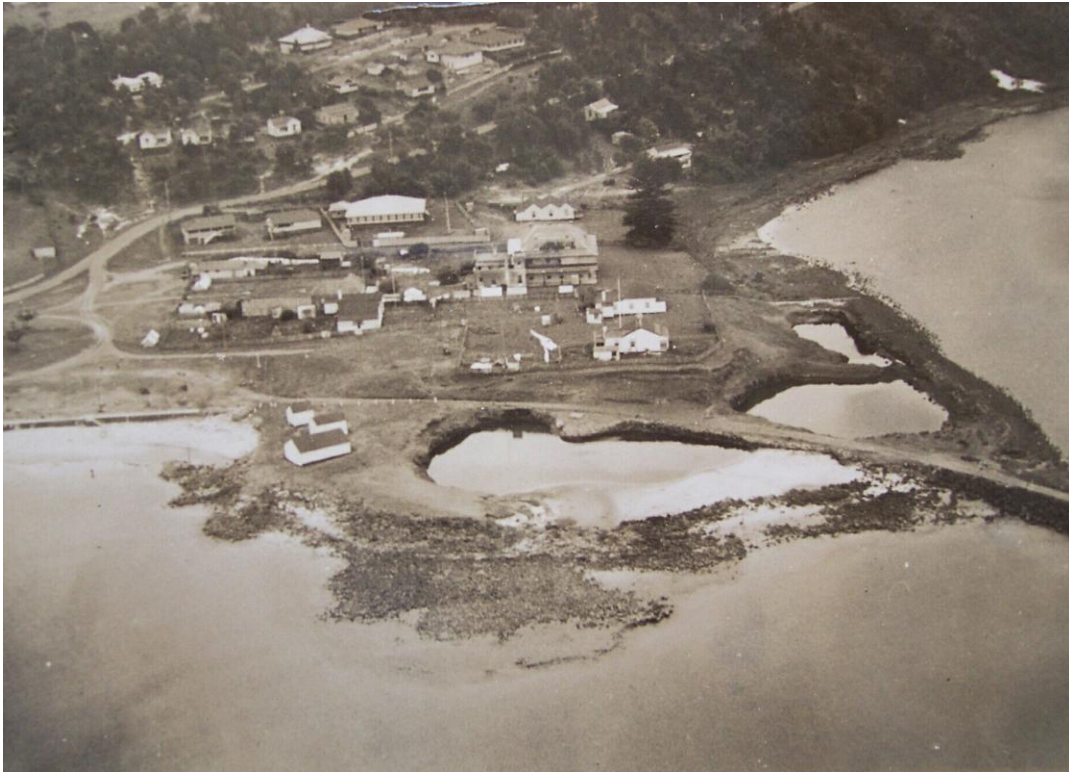
Shaws Bay, showing buildings associated with the Ballina Pilot and 'quarry holes' formed by the removal of columnar basalt to construct the Ballina breakwall. Image courtesy of BSC records.
