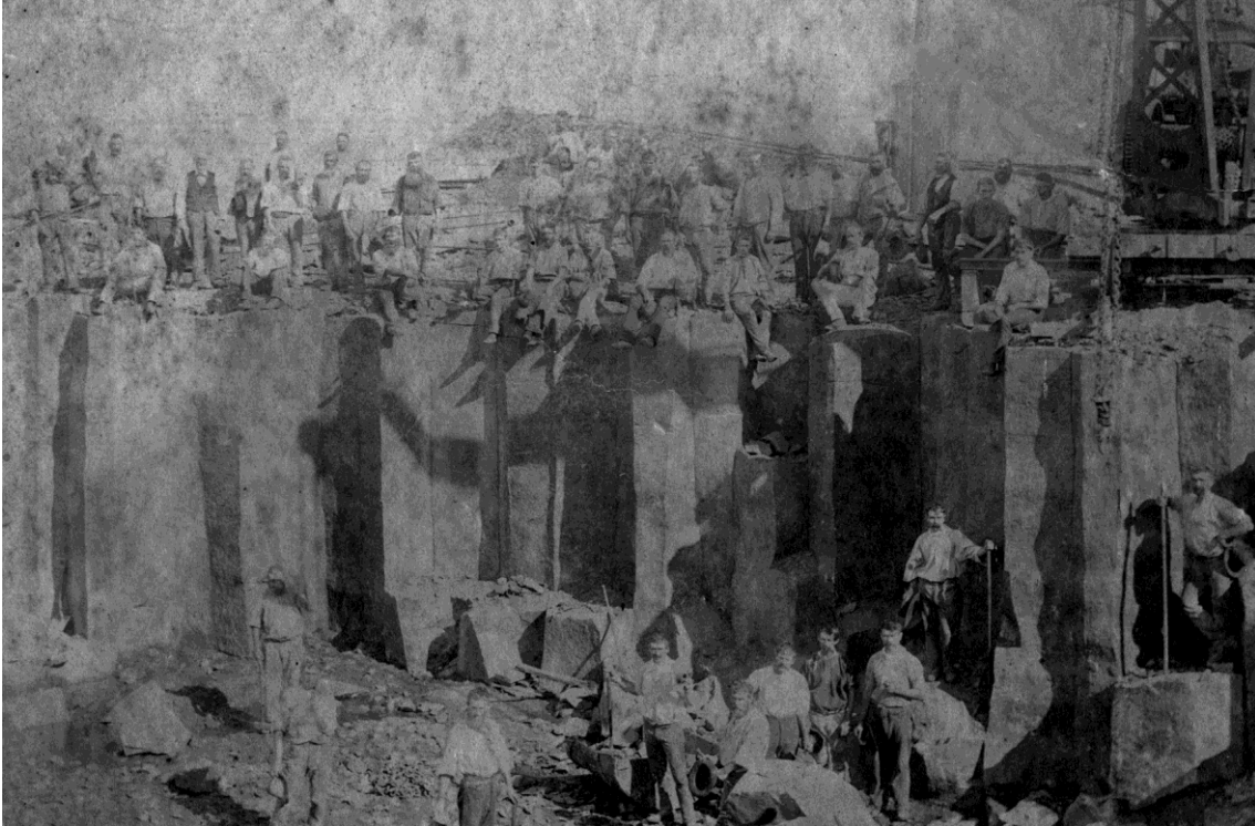
Quarrying columnar basalt for construction of the Ballina breakwall. Image taken by photographer Joseph Check, 1890s, and courtesy of Richmond River Historical Society.
