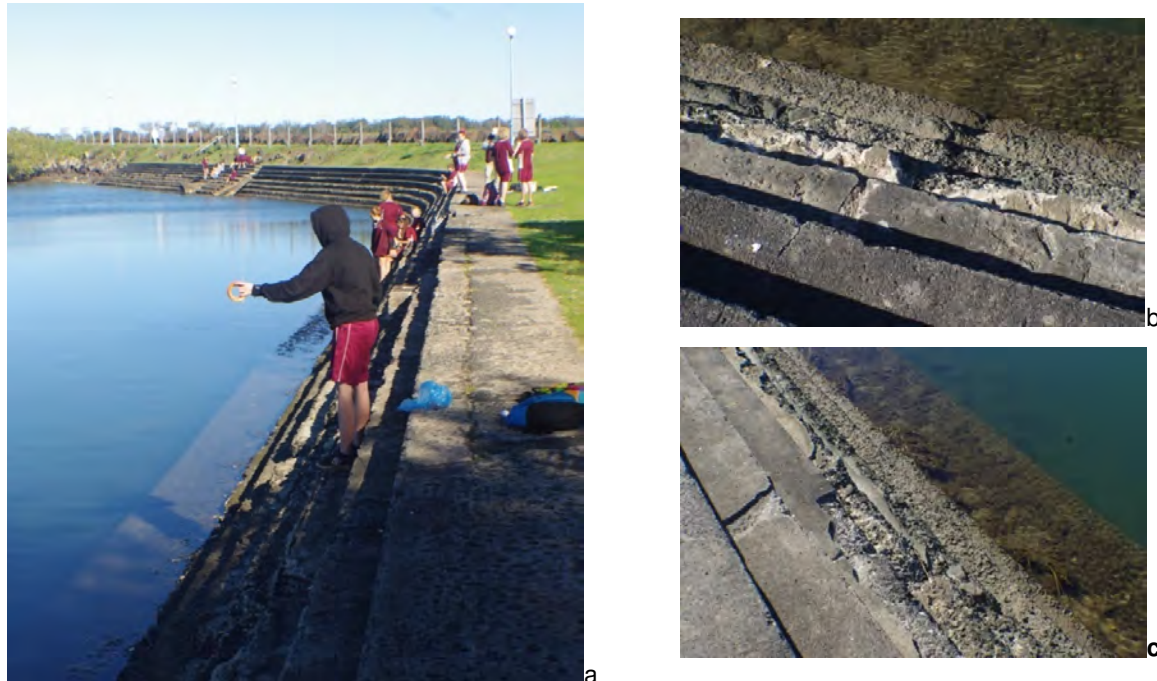
Figure 20: Training wall concrete steps
