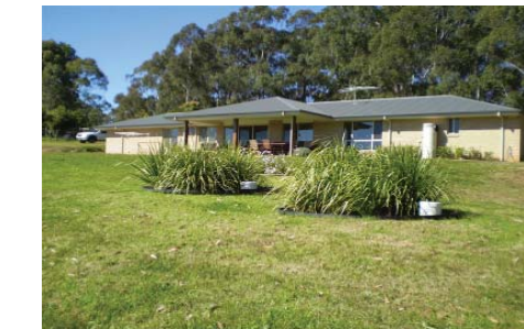
Photo courtesy of Midcoast Reedbed Wastewater Systems
