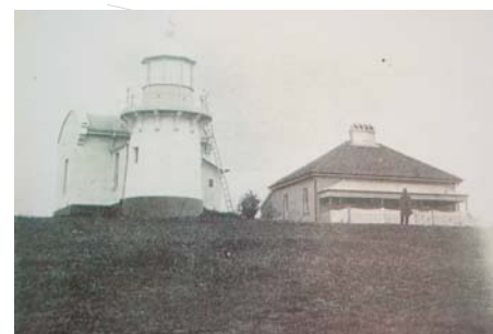
(b) 1902 Richmond River Lighthouse and Lighthouse Cottage
