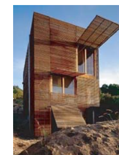
(e) 'Open' Breamelea House, Architect: Sean Godsell
