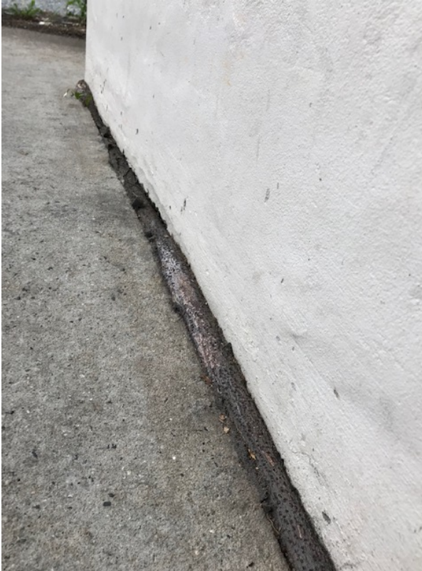
Fig tree root between slab and wall B. Branch 04/02/2020
