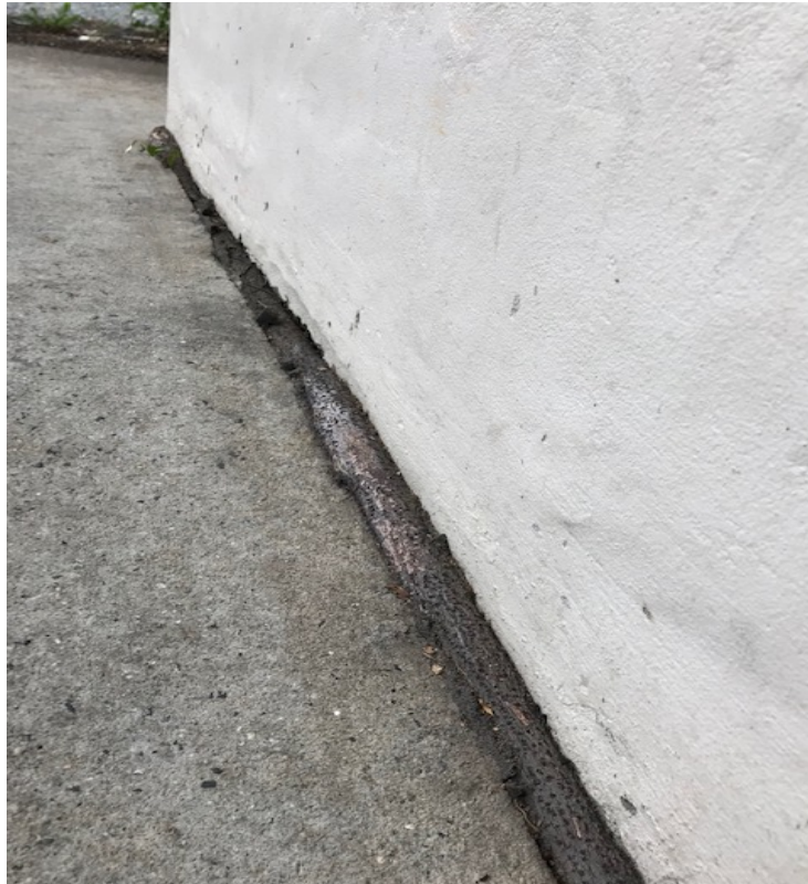
Fig tree root between slab and wall B. Branch 04/02/2020
