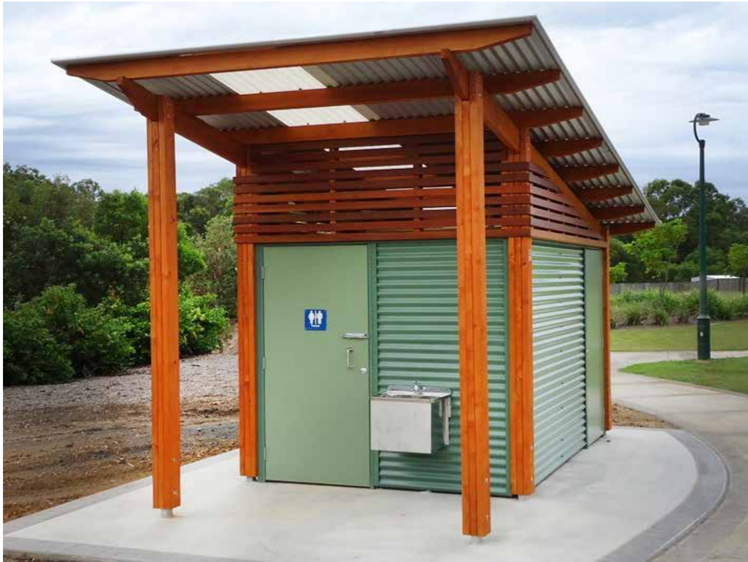
LANDMARK TOILET BLOCK (POTENTIAL AMENITIES) (NOT PART OF THIS STAGE) (COLOUR SELECTION IN CONJUNCTION WITH SITE FURNITURE TO BE CONFIRMED)
