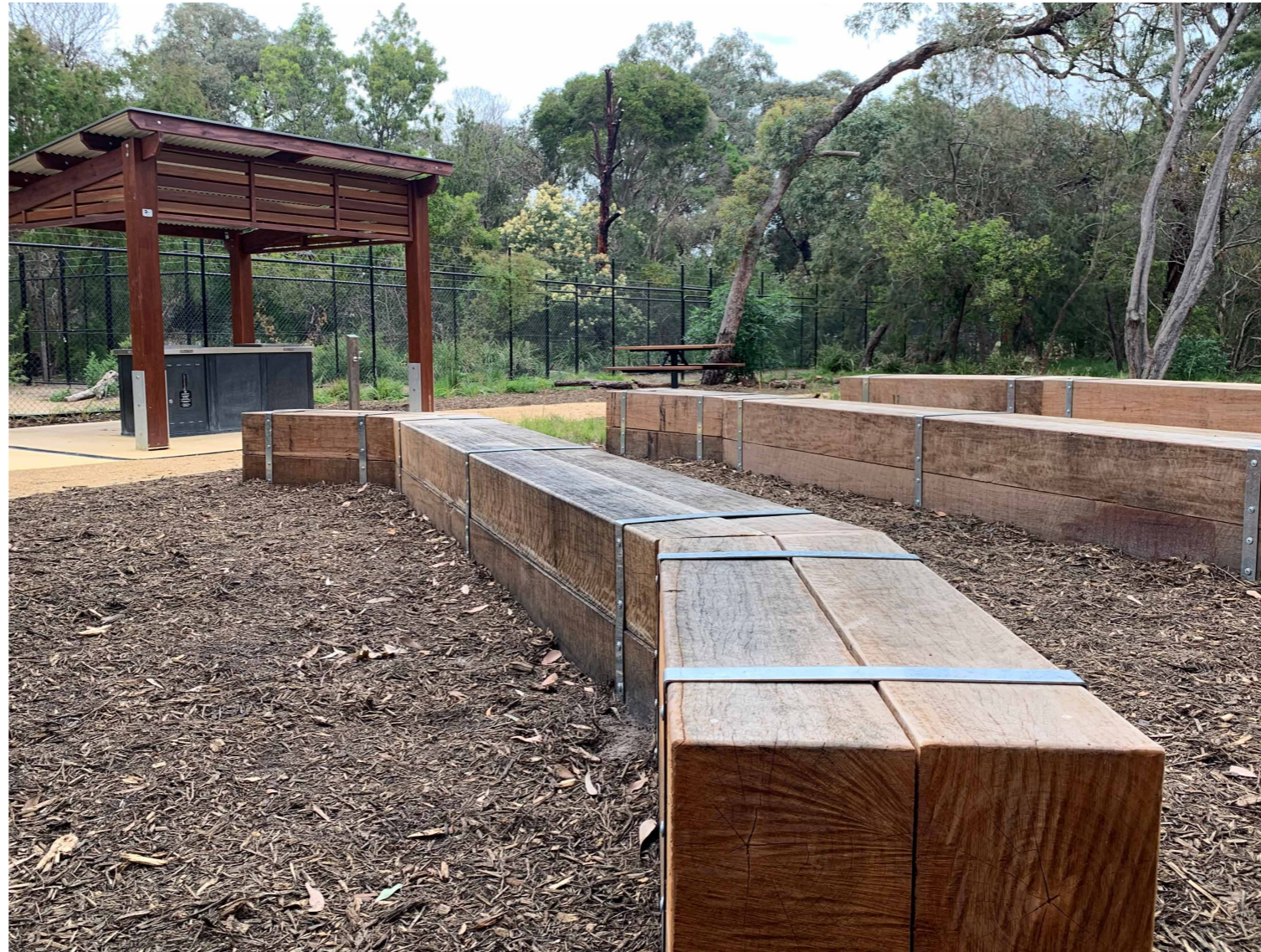
SQUARE TIMBER SEAT (450X450MM) (COUNCIL SUPPLIED TIMBER - MAY BE 1X450MM SQUARE PIECE)
