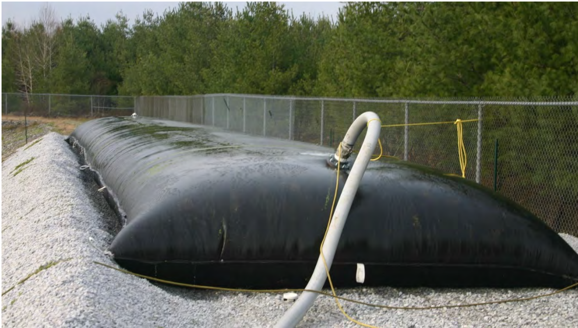
Plate 5. Example of geobag containment
