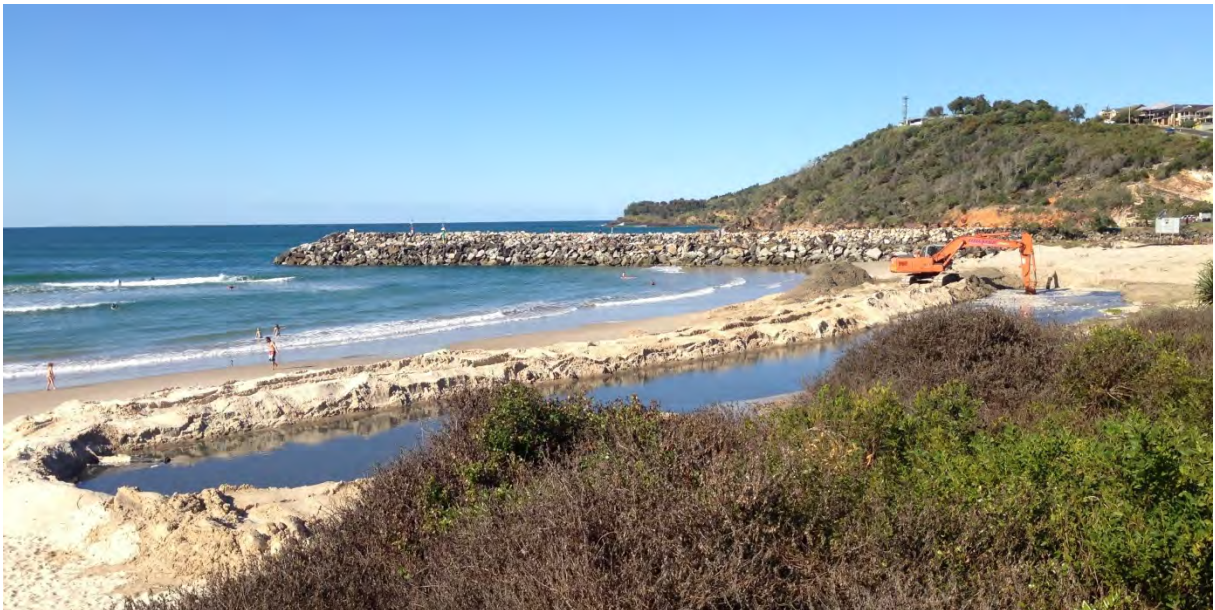
Plate 3. Large scale bunded beach area receiving dredged sand
