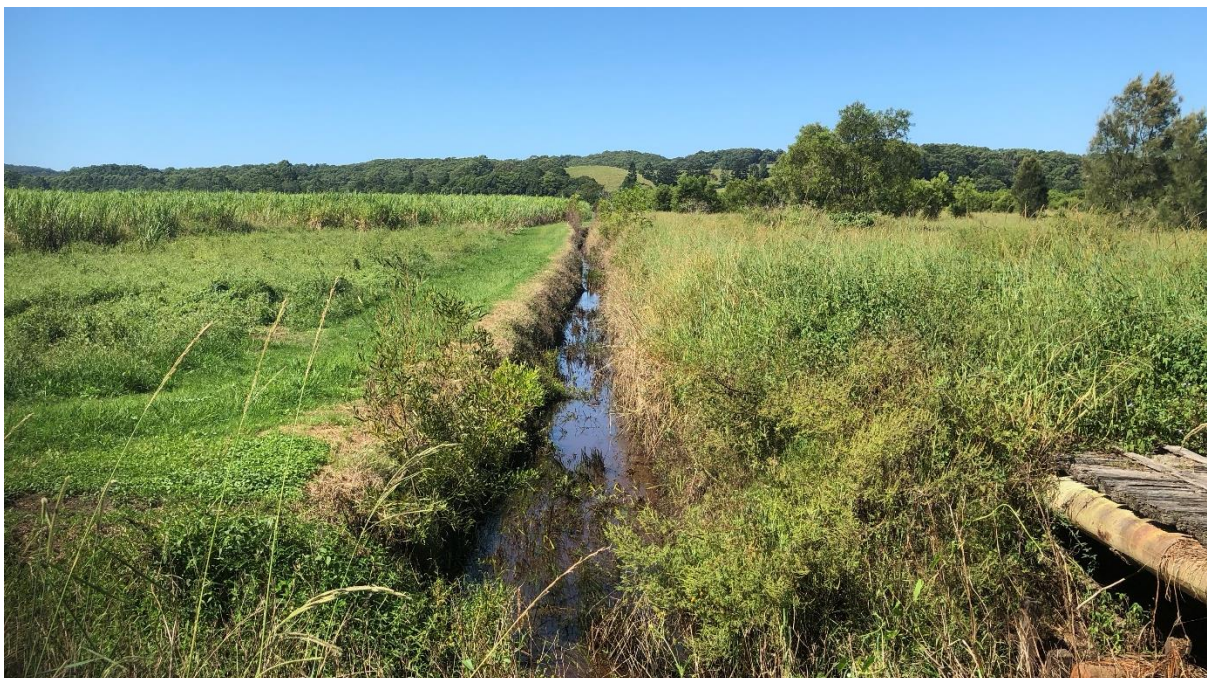
North Creek – linear drain in upper catchment (2018)
