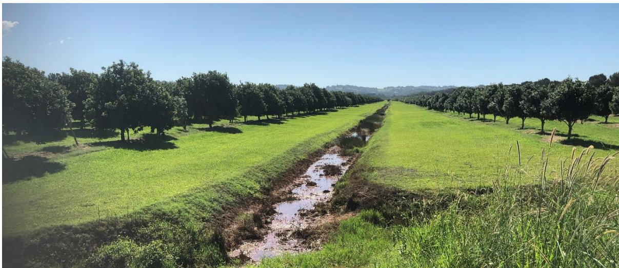
North Creek – drainage channel in upper catchment (2018)
