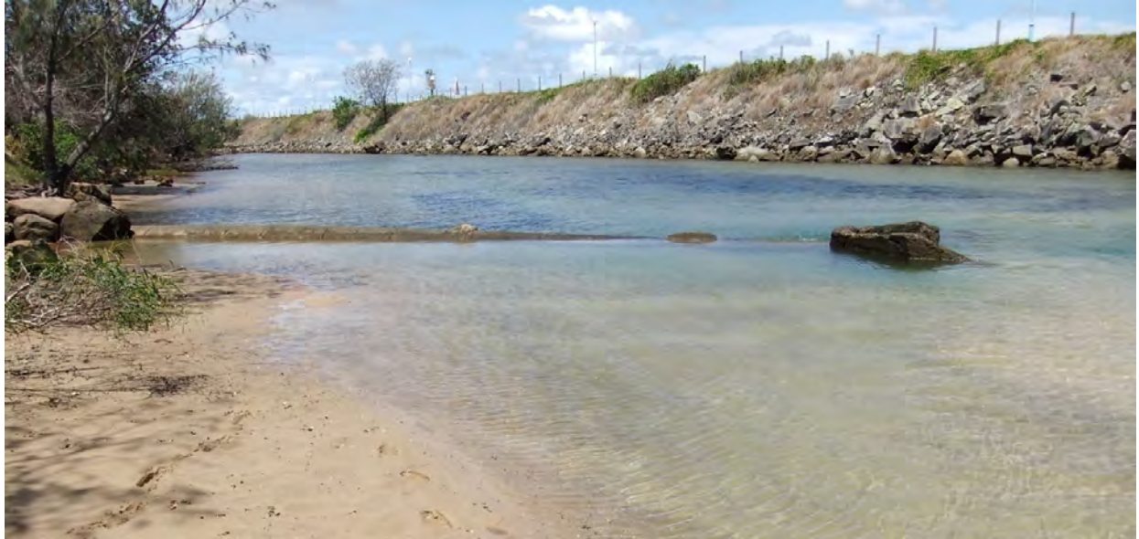
Figure 14: Shoreline recession indicated by location of stormwater outlet in the East Arm
