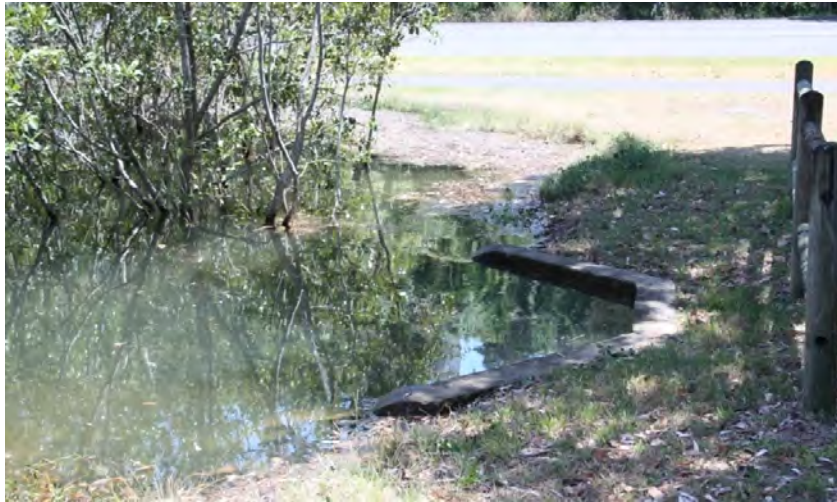
Figure 19: Tidal inundation of stormwater drain (January 2014)
